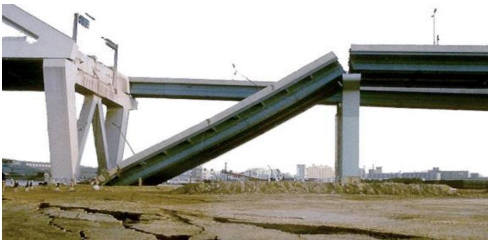
Figure 2. 1995 Hyogo-Ken Nanbu earthquake. Nishinomy-ko bridge
