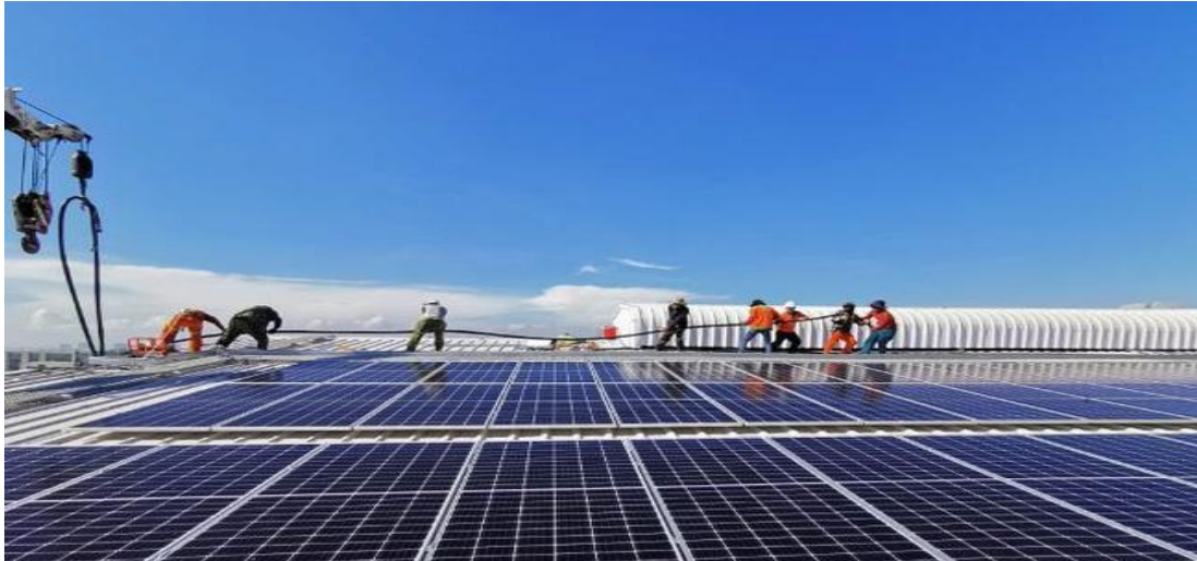
Figure 2: The installation process of the Koyosh panel.
