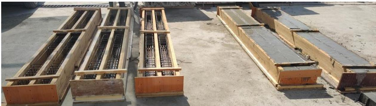
**Fig. 7. Forming concrete beams**
