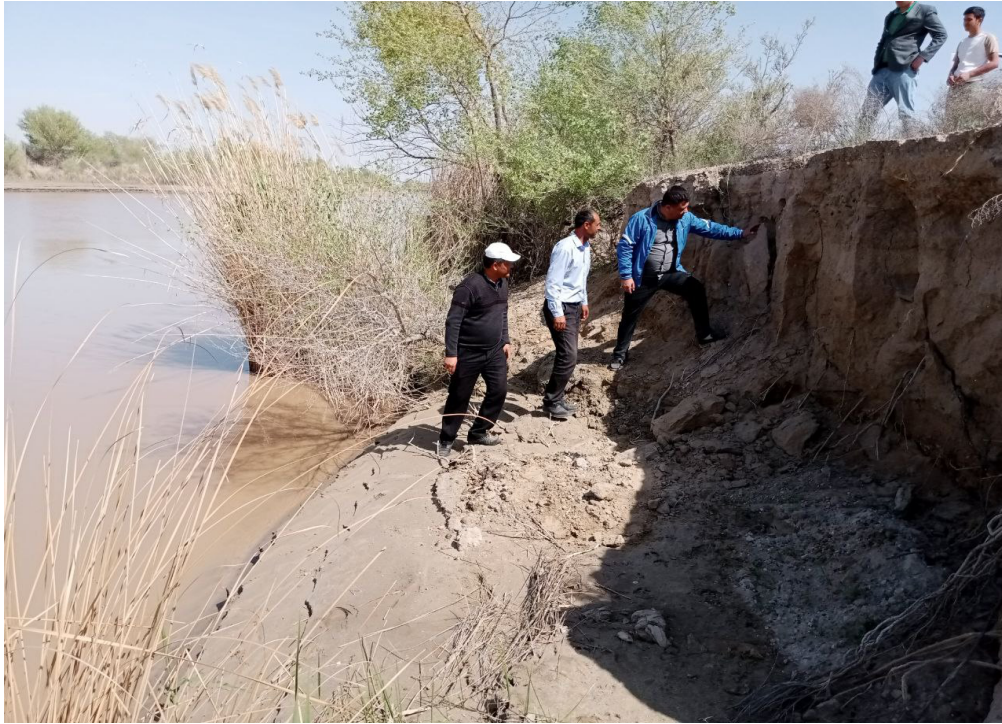
Figure 1. The condition of the right bank erosion of the Amu-Bukhara Machine Canal at PK 950 station
